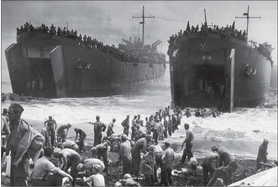
U.S. troops build sandbag piers to speed up the unloading of tanks, supplies, and equipment from two landing ships—the LST-22 and LST-206—during the Battle of Leyte in the Philippines on October 1, 1944. FPG/Hulton Archive/Getty Images
