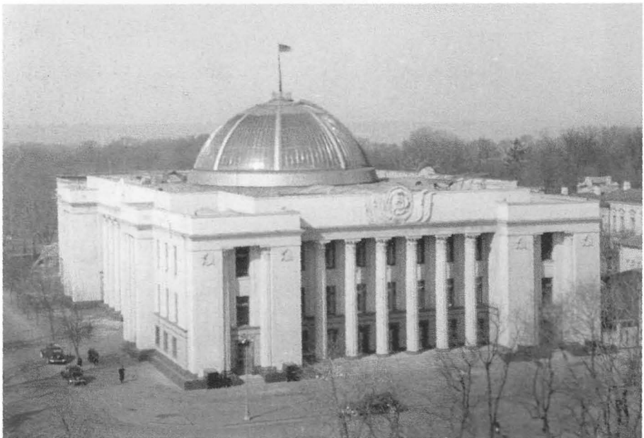
9 The Praesidium building of the Supreme Soviet of the Ukraine in Kiev. The architect, V. I. Zabolotni, was awarded a Stalin Prize for the design, completed in 1939. In cities all over the Soviet Union the new built environment was intended as a monument to the Stalinist utopia.
