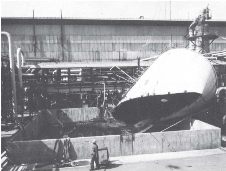
FIGURE 5-1 Corrosion and missing holding-down bolts caused this tank to fail at the base instead of the top.
