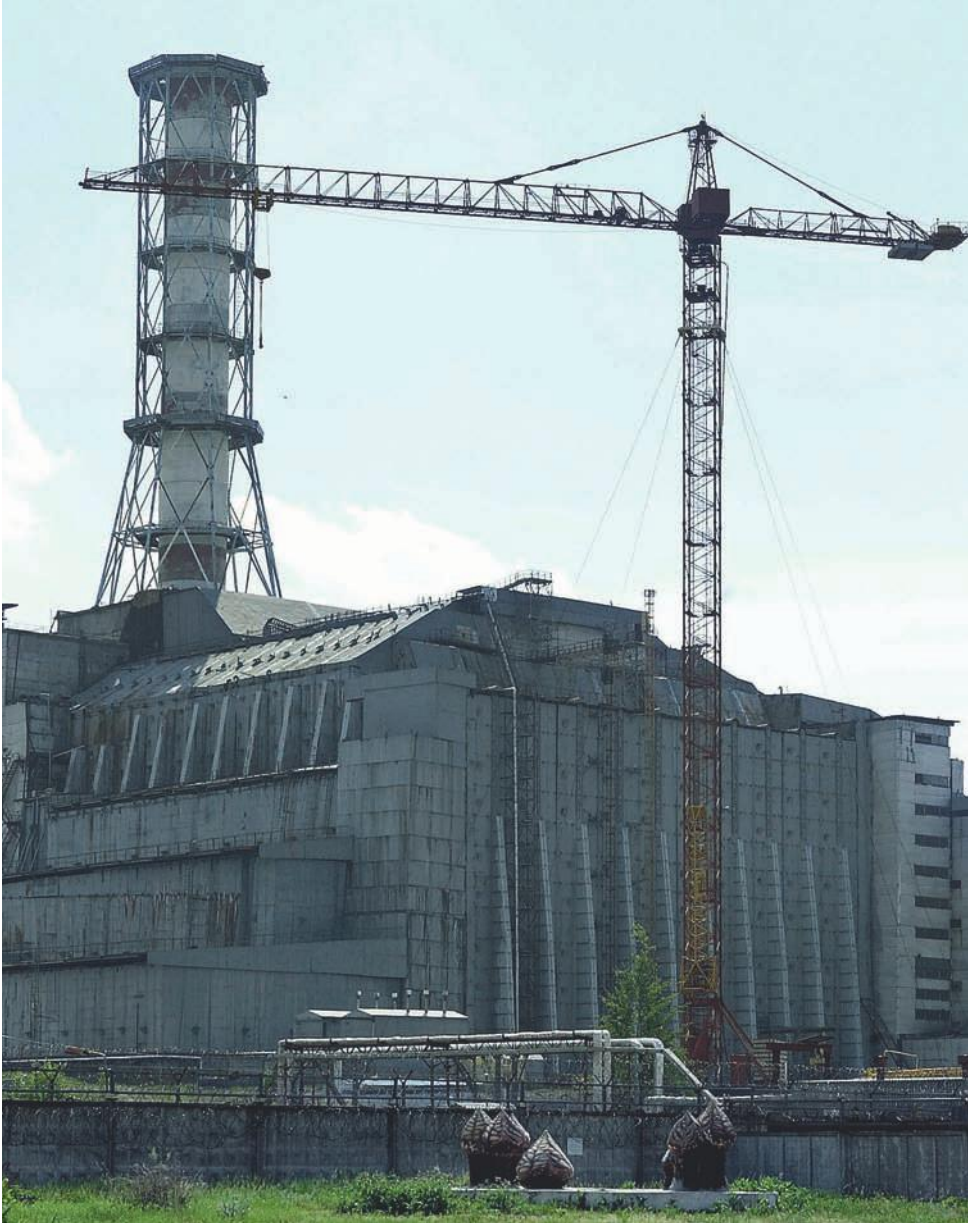
The Sarcophagus, a concrete and steel structure, covers the damaged reactor at Chernobyl.
