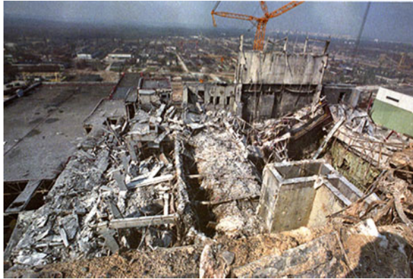
Fig. 8.3 Chernobyl #4 reactor accident
