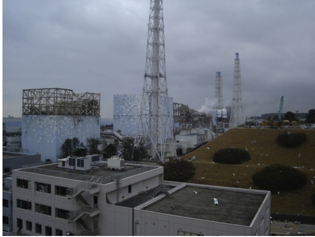
Figure 3.8 Units 1, 2, 3 and 4 of the Fukushima Dai-ichi NPP after a hydrogen explosion in Unit 3 on 15 March 2011. (Source: Reprinted with permission of TEPCO)
