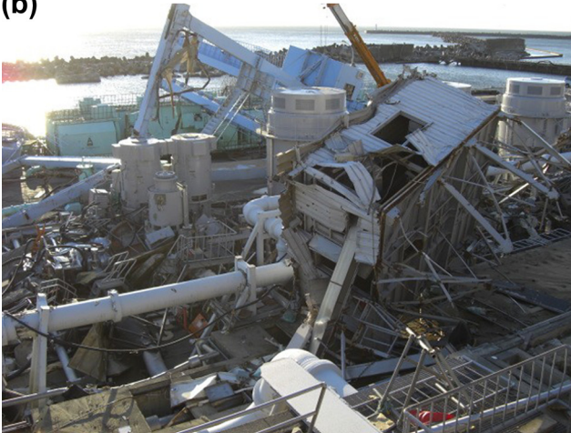
Figure 3.3 Tsunami waves in front of the Fukushima Dai-ichi NPP on 11 March 2011 (a), and destroyed equipment of the seawater pump area (b). (Source: Reprinted with permission of TEPCO)
