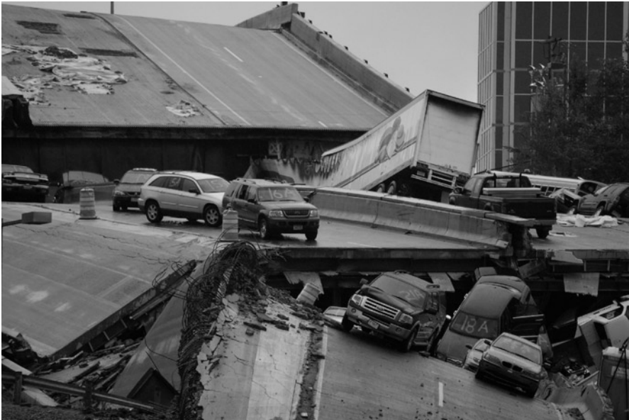
Fig. 9.3 Collapsed Interstate 35 Bridge in Minneapolis, August 31, 2007. (Source: Wikimedia)
