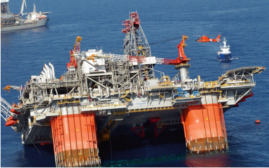
Fig. 2.9 The U.S. Coast Guard reported on July 12, 2005: “Thunder Horse, a semi-submersible platform owned by BP, was found listing after the crew returned. The rig was evacuated for Hurricane Dennis.” This almost $1 billion platform was nearly sunk by an incorrectly plumbed 6-inch. pipe valued at just a few dollars. Then there were problems with welds in the subsea pipes and manifolds. Their replacement cost and 3 years of production delays might have been as high as another billion USD. (Image Source: USCG photo by PA3 Robert M. Reed, displayed in Wikipedia)
