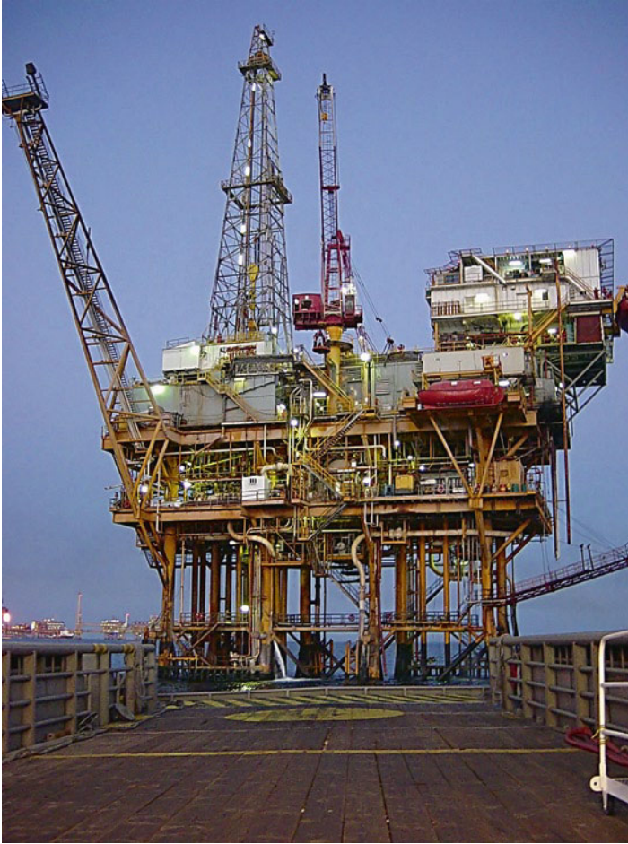
Fig. B.I A fixed platform in the Gulf of Mexico. (Source: www.digitaljournal.com )
