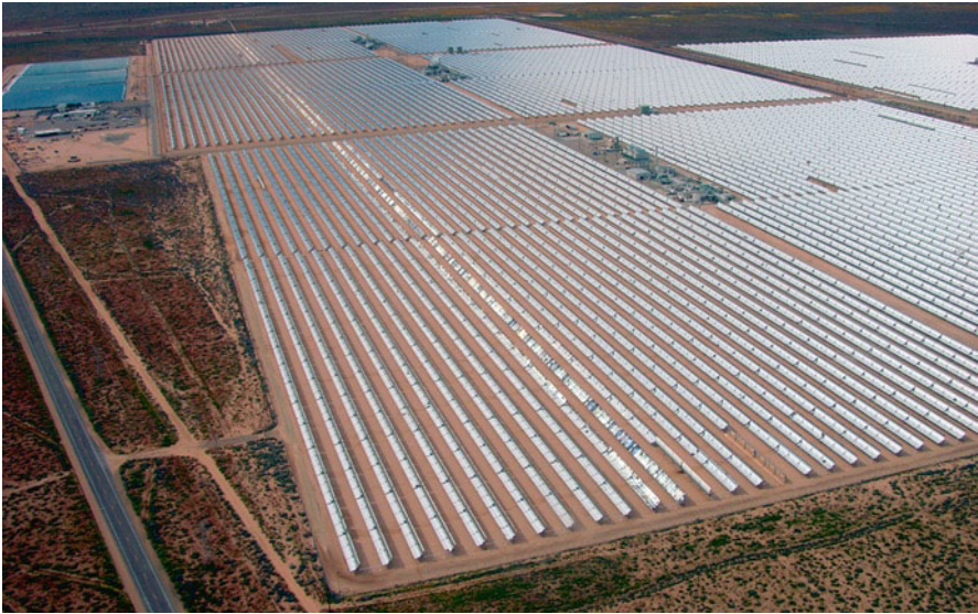
Fig. 9.2 The Nevada Solar One plant, a solar energy concentrator that covers 1.6 square kilometers of land and provides 15 megawatts of electricity on average. Its vastness can only be appreciated from the air. The figure of 15 megawatts is obtained by dividing the number of kilowatt-hours actually sold in one year by the number of hours in a year. At today's power requirements, this plant can serve 1,440 people on average. We would need to build 211,000 such plants to generate 250 kWh/p/day, which is current U.S. consumption
