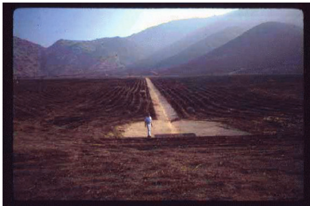
FIGURE 5.9 Worker standing on surface drainage gutter and drain inlet basin in the southern part of Zone 1, facing northeast. 25 K at Stringfellow site. Photo credit: U.S. Environmental Protection Agency. http://yosemite.epa.gov/r9/sfund/r9sfdocv.nsf/3dc283e6c5d6056f88257426007417a2/701f424f17ca525d8825700700754b3b!OpenDocument [accessed January 4, 2012].
