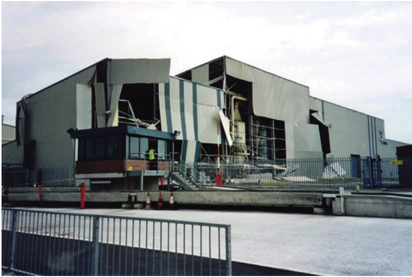
FIGURE 3.2 Aftermath of wood dust explosion. Taken from http://www.hse.gov.uk/woodworking/fire.htm .
