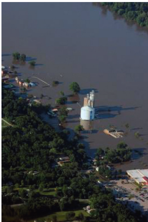
FIGURE 5.1 Aerial of farm structures flooded by the Mississippi River at La Grange, Missouri on June 20, 2008. Photo by J. Augustino. Source: Federal Emergency Management Administration, 2011.
