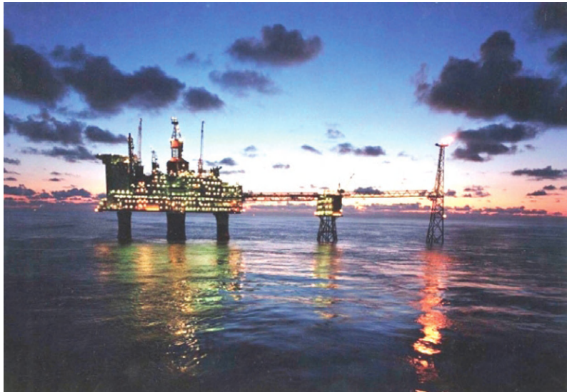
FIGURE 8.18 Carbon dioxide that is produced at the Sleipner natural gas complex off the coast of Norway is removed and pumped into the Utsira Formation, a highly permeable sandstone. In this case, the sequestration cost is less than the Norwegian carbon emission tax. Photograph is courtesy of Øyvind Hagen, Statoil.
