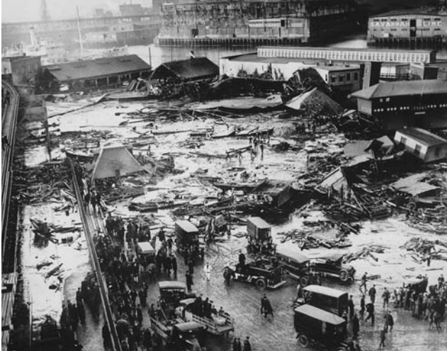
With the wreckage of the collapsed Purity Distilling Company storage tank visible in the background, tons of sticky molasses coagulate on the streets of Boston. (Boston Public Library)
