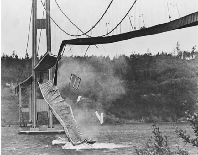
In one of the most stunning disaster pictures ever taken, the Tacoma Narrows suspension bridge plunges into the water amid high winds. Note the automobile moments before it plummeted. ( Library of Congress )
