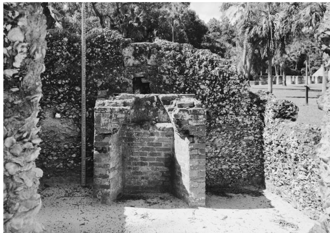
Tabby construction in ruins of Kingsley plantation, Jacksonville, Florida. (Library of Congress.)
