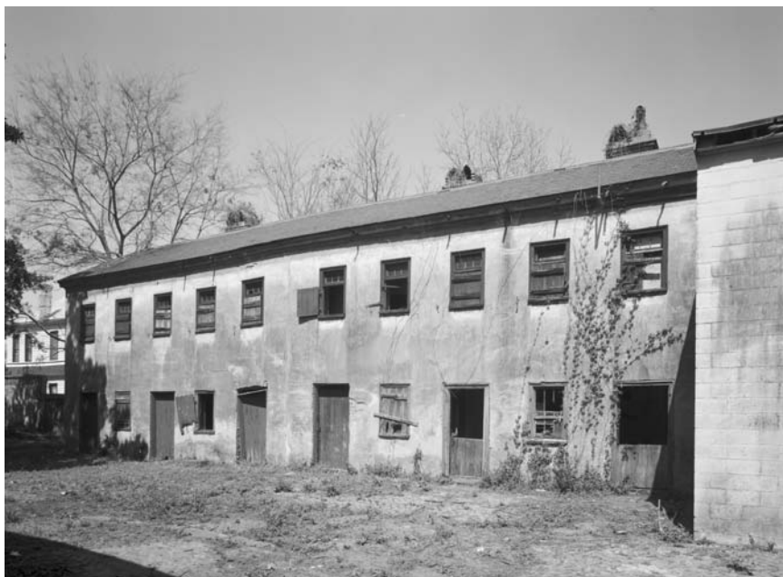
Robinson-Aiken slave building and kitchens, Charleston, South Carolina. (Library of Congress.)
