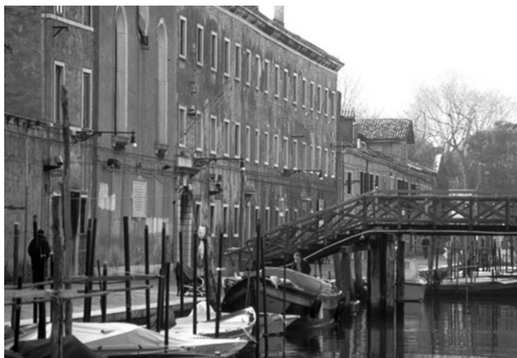
Figure 4.2 Side view of the bridge leading to the Convertite . Photo taken in 2002
