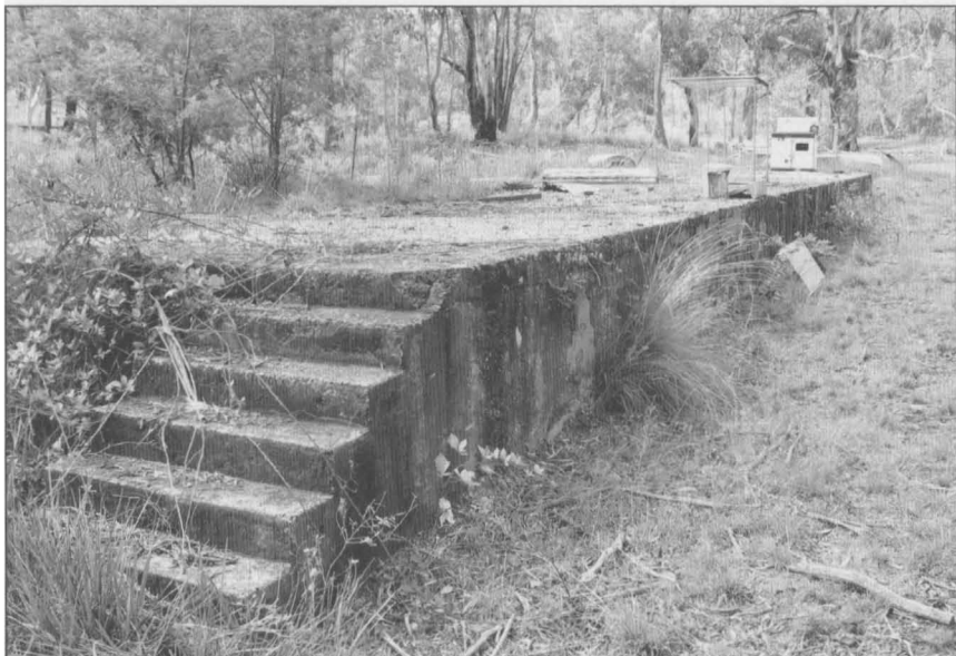
Phosgene Shed Foundations Today.
