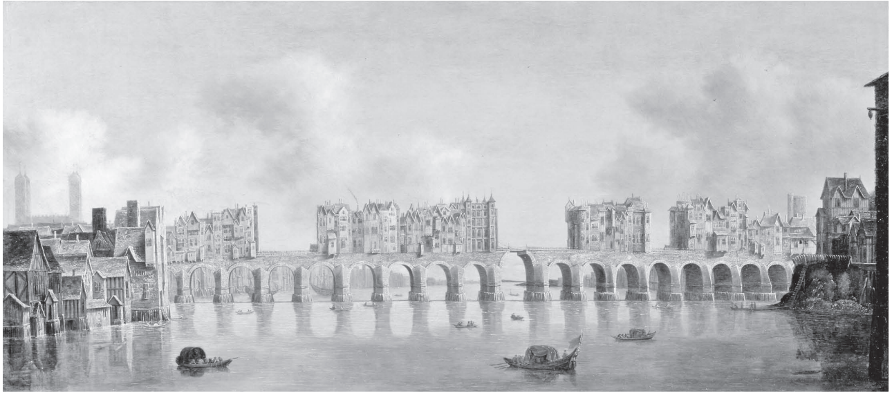
FIGURE 14 A view of London Bridge as it appeared in c.1632, by the Dutch artist Claude de Jongh. The narrow openings between the stone pillars are clearly visible, and it was the hazards caused by the strong currents swirling through the gaps at high tide that delayed Elizabeth's passage to the Tower in March 1554, so saving her life.
