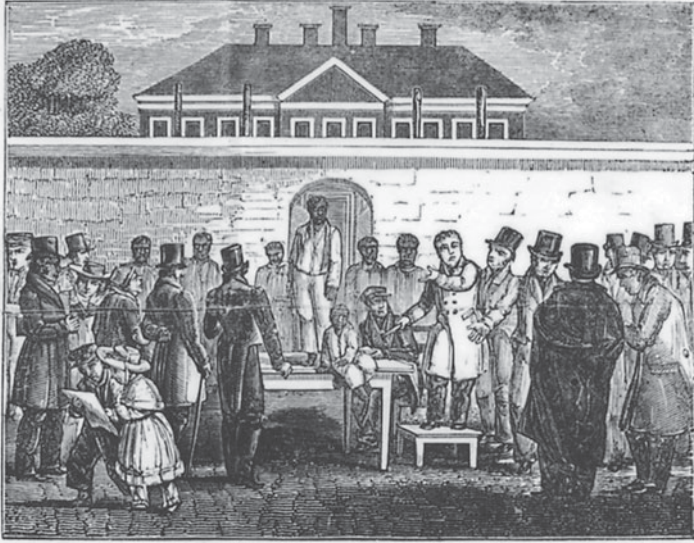
Illustration of free people of color being sold into slavery in Washington, DC, for failure to pay their jail fees. From the broadside “Slave Market of America” published by the American Anti-Slavery Society in 1836. Courtesy of the Library of Congress.
