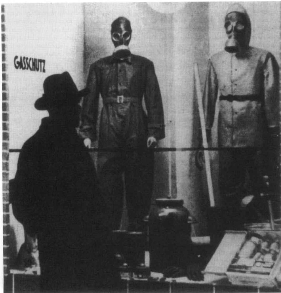
Mannequins with chemical protective gear in a German window display, March 1939
