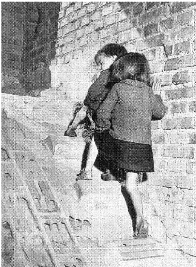
Two children climb out of the cellar into their gutted home.
