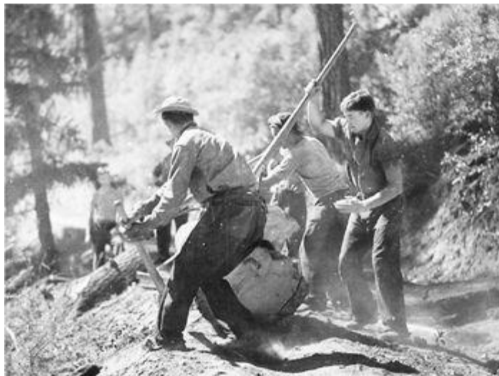
Civilian Conservation Corps (CCC) crew at work in Idaho’s Boise national forest.
