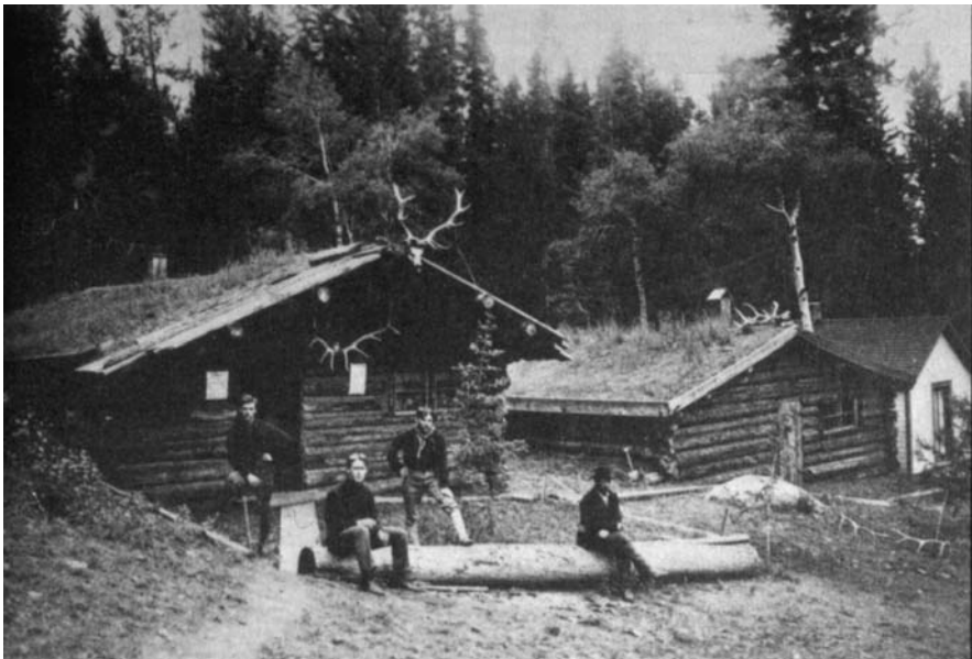
Fig. 1.8 Soldiers stations, such as this one at Tower Falls, were established throughout the park to protect the park's attractions in the summer and resist poachers in the winter (NPS Photo, photographer unknown)
