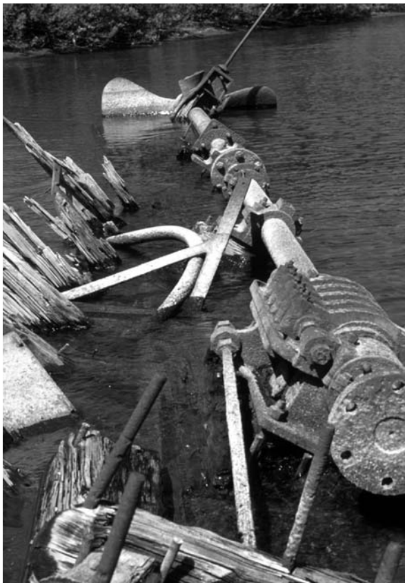
Fig. 2.56 View west of E. C. Waters' propulsion system. The engine bed is in the foreground, the thrust bearing is in the middle foreground and the propeller shaft and the propeller is in the background. NPS photo by John Brooks
