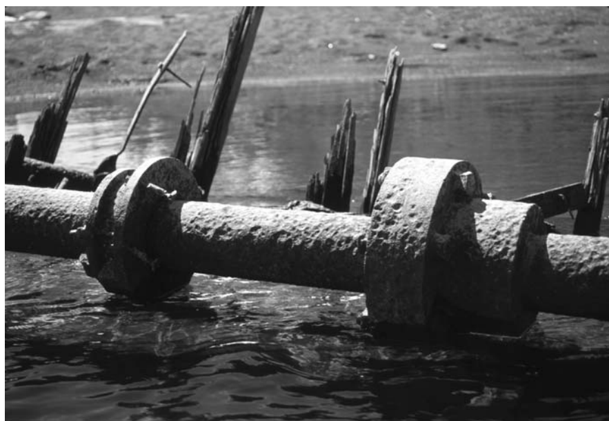
Fig. 2.60 View southeast of after bulkhead stuffing box and gland ( left ), and propeller shaft coupling ( right ). NPS photo by Brett Seymour
