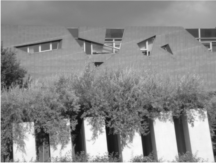
Figure 8-8. Exterior, view of Peace garden with Jewish Museum Extension beyond. Photographed by Frank H. Weiner.
