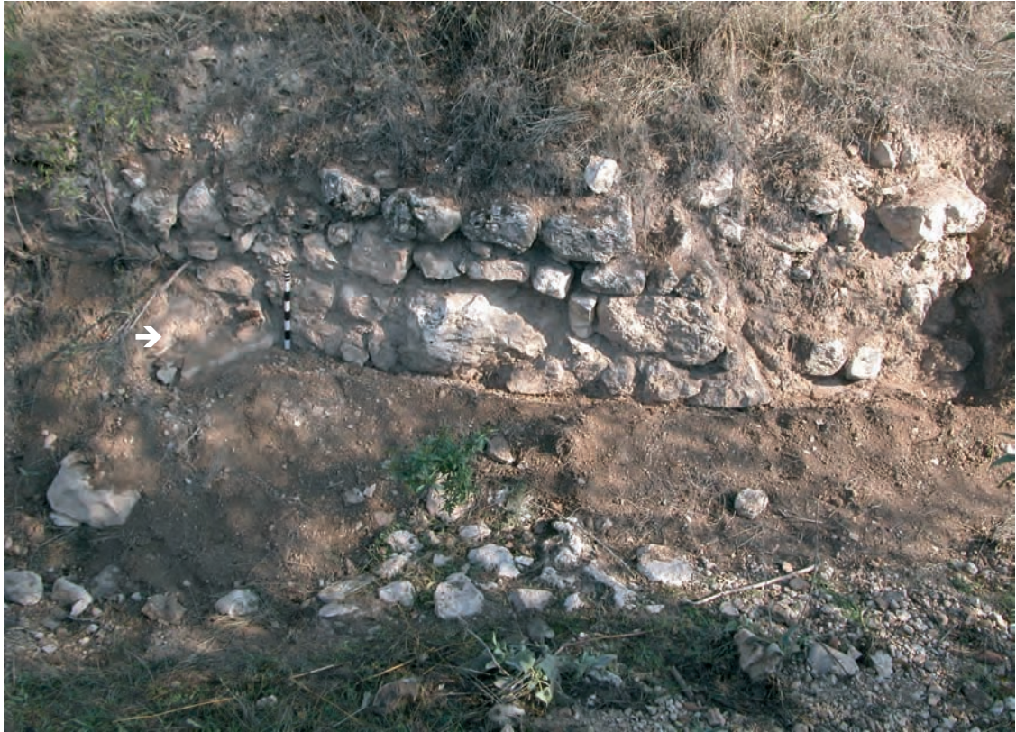
Fig. 10.14 Pepouza central part: water pipe in northern embankment of low-lying road (left of scale stick)
