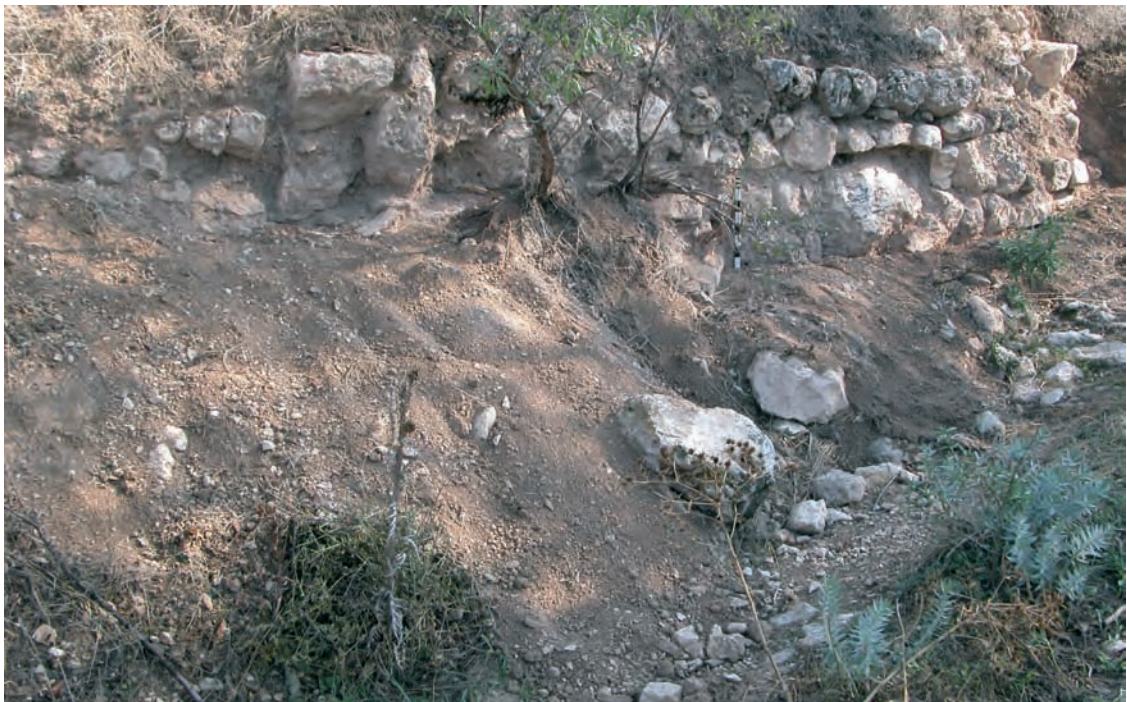
Fig. 10.15 Pepouza central part: water pipe in northern embankment of low-lying road (left of scale stick)
