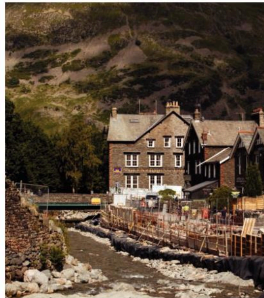
Fig. 4.33 New food defences being built, Glenridding, Cumbria
