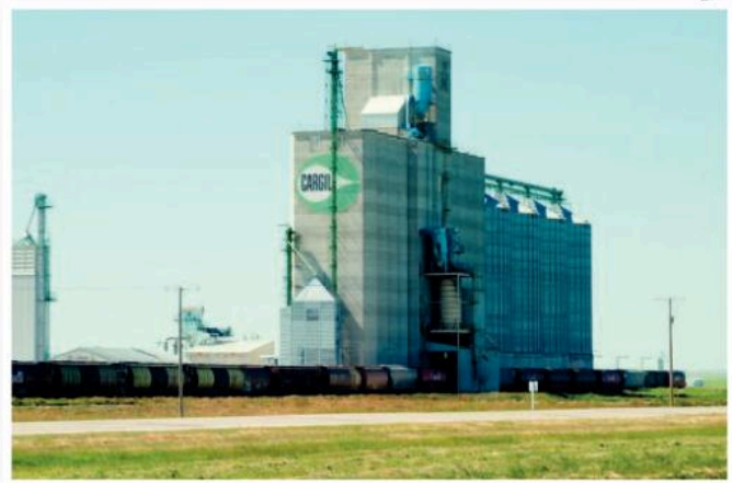
Fig. 9.20 A grain elevator
