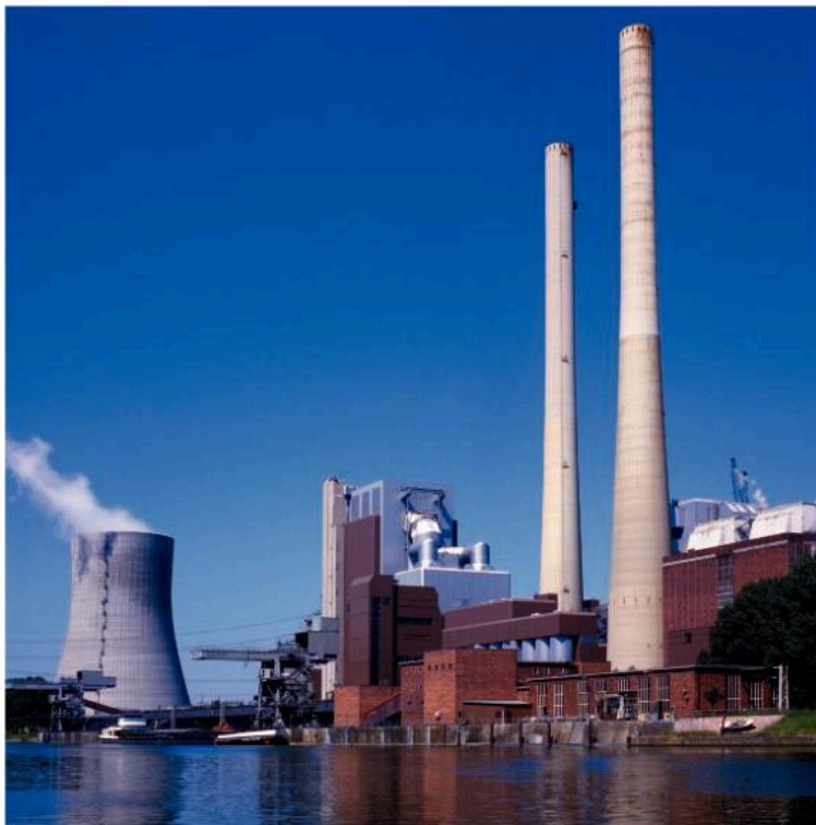
Fig. 11.29 The Heilbronn coal-fired power station on the River Neckar. Notice the river to provide cooling water (and sometimes transport for coal). Also notice the tall chimneys to disperse oxides of nitrogen and sulfur dioxide, together with the cooling tower in the background.
