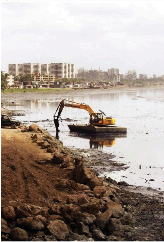
Fig. 2.53 Dredging along the Mithi River helps the water to flow faster to the sea (along with all its waste)
