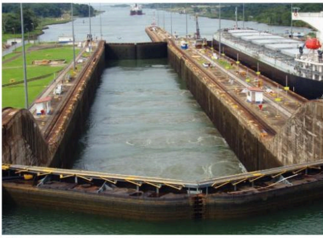
Fig. 7.41 Two parallel sets of locks along the Panama Canal lead into Lake Gatun
