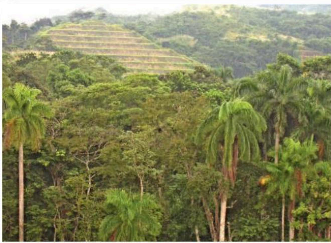
Fig. 7.42 The far hillside was excavated for the third set of locks (it has to be terraced to prevent landslides)
