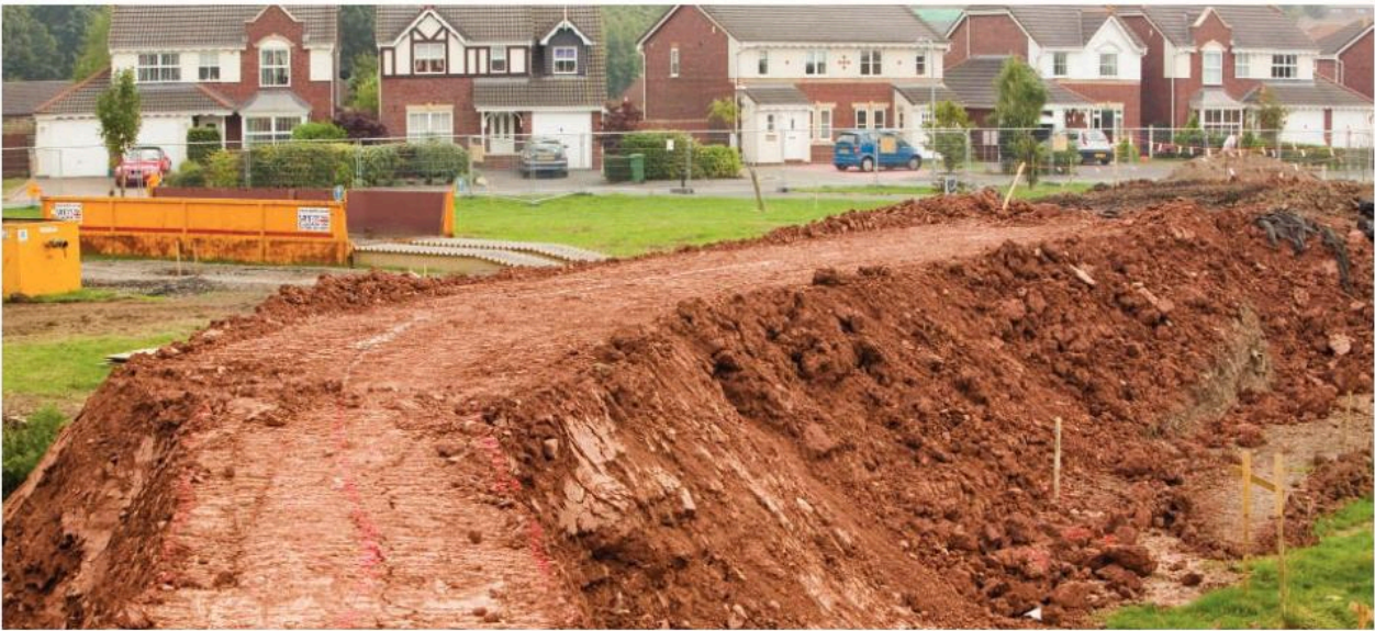
Fig. 4.32 Building new flood defences in Carlisle, Cumbria
