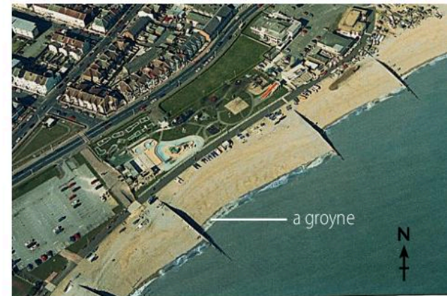
▲ The groynes stop the beach being carried away.
