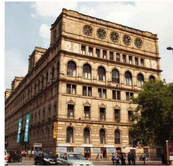
▲ This was once a cotton warehouse. The merchant was doing well! It opened in 1856. Today it's an hotel.
