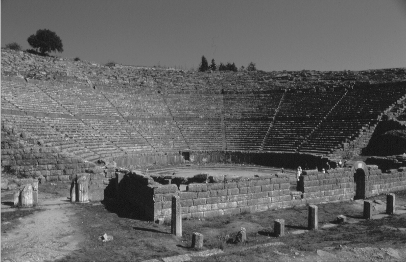
Figure 7.4 Dodona, Epeiros: the theatre constructed originally under king Pyrrhos of Epeiros (297–272 BCE) and rebuilt by Philip V of Macedon soon after 219 BCE. A building programme begun early in the fourth century, with the construction of the first temple of Zeus, culminated in the theatre. Copyright: C. B. Mee.
