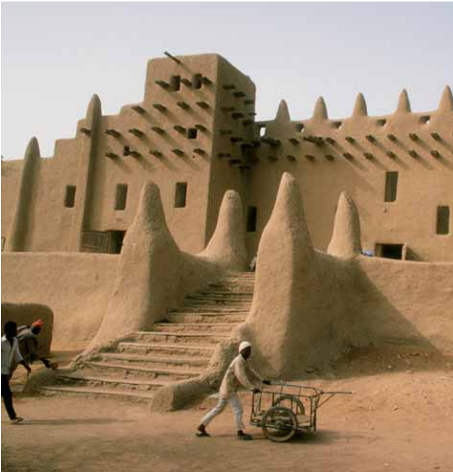
The Grande Mosque, in Djenne, Mali, is the world's largest mud brick structure. It was originally built in the 13th century by Koy Konboro, Djenne's first Muslim ruler. (Corbis)
