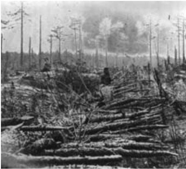
Confederate entrenchments near Spotsylvania Court House, showing felled trees placed in trenches (Library of Congress)
