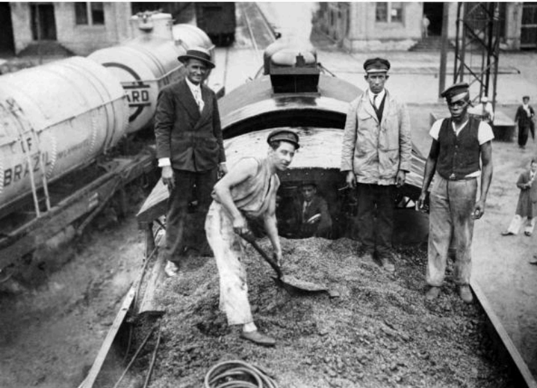
▲ Mixing coffee into tar to be used in building new roads and highways
