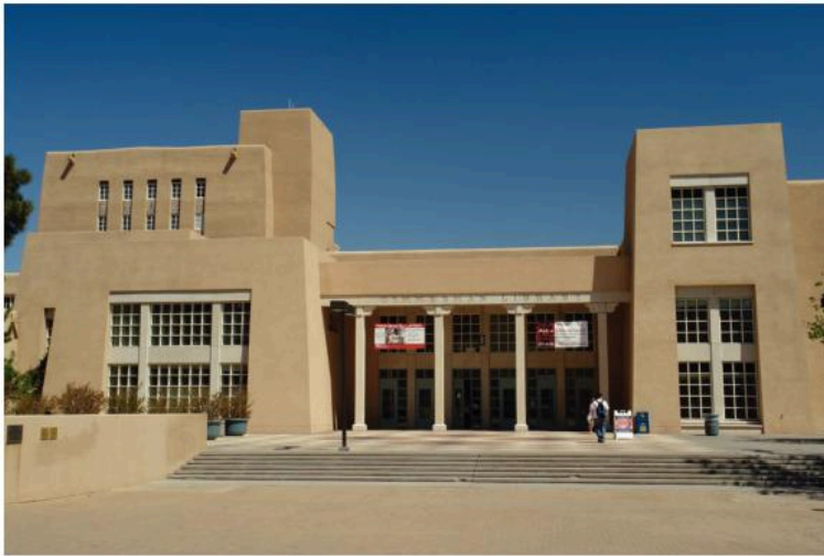
▲ The Zimmerman Library at the University of New Mexico was a New Deal project designed by architect John Gaw Meem
