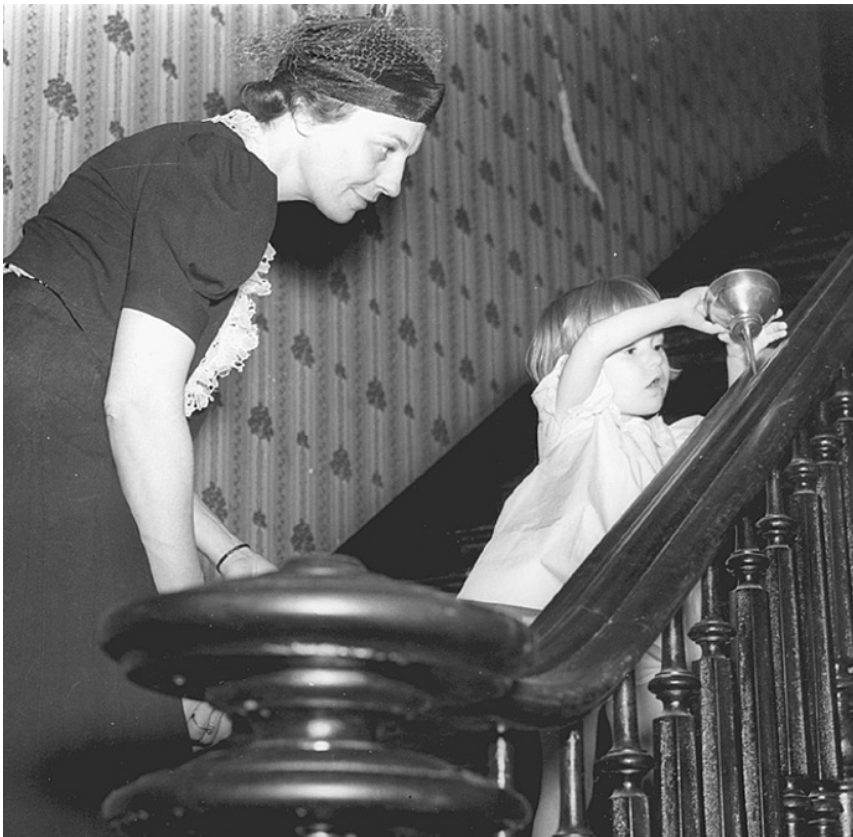
Figure 10.4 Free Nursery School at 122 Nolan Street, San Antonio, a WPA project. Sallie Schurcard, as a child, oiling a staircase railing as an attendant looks on. Source: The San Antonio Light Collection , University of Texas at San Antonio Libraries Special Collections, Institute of Texan Cultures at San Antonio (MS 359: L-2057-E).
