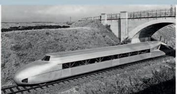
**Zeppelin train** Built by Franz Kruckenberg of Hannover the *Schienenzeppelin* only had two axles and was designed to carry 40 passengers.
