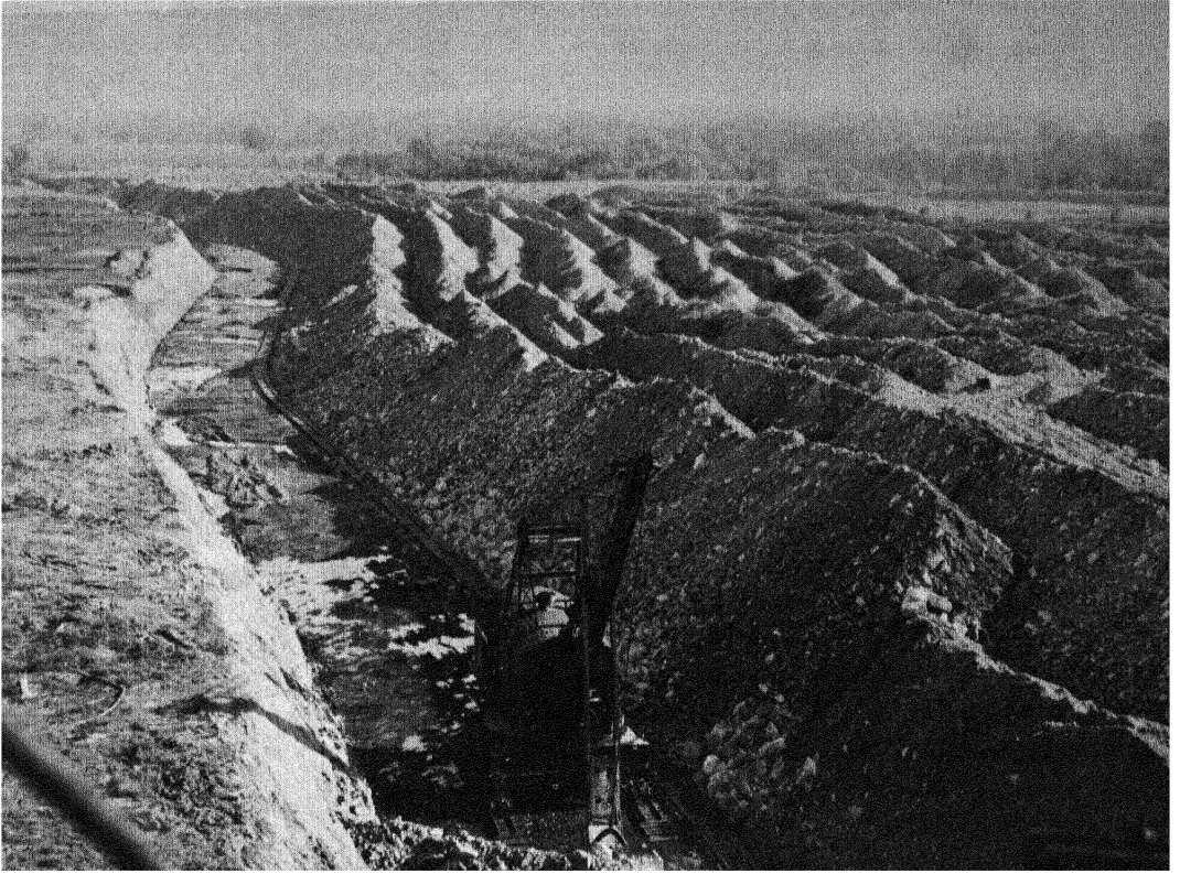
FIG. 19.2 Giant furrows turned by power shovels in the process of strip mining in southern Illinois. The 4-ft-thick bed of coal exposed in the bottom of the trench will be mined out before the next furrow is turned.
