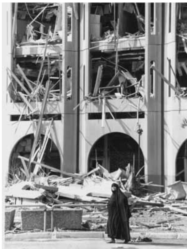
A typical scene of the destruction in Baghdad during the Gulf War.
