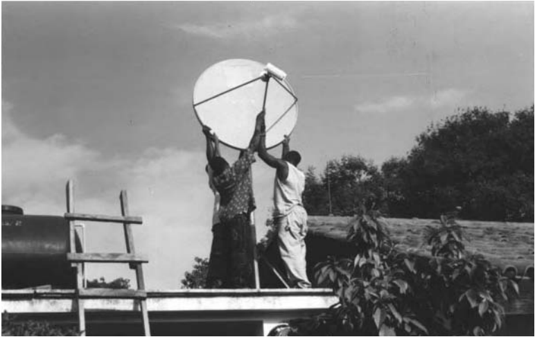
Technicians installing the VSAT
