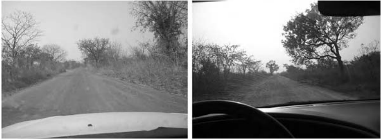
Shots of the road layout to some of the regions reached by the Project's staff
