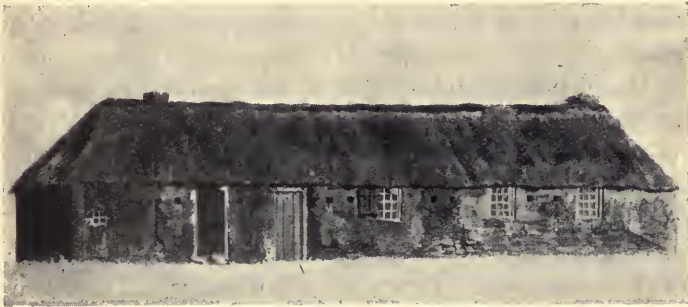
GUARD HOUSE, GRAHAMSTOWN
