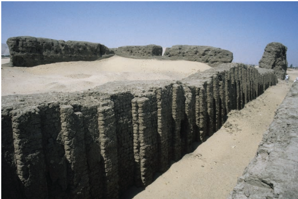
Plate 1 The mud-brick funerary enclosure of King Khasekhemwy at Abydos (Shunet ez-Zebib) (Second Dynasty). © Toby Wilkinson.
