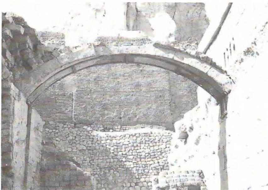
Pl. 51 A (Top): Dendera enclosure wall.
