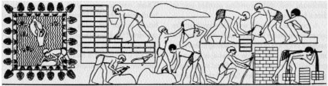
A scene from the tomb of Vizier Rekhmire (c.1450 BC), showing the production of mud bricks. Alluvial mud is mixed with water (left) and then packed into wooden molds. When lifted, the molds released the bricks so that they fell onto the ground where, arranged in long rows, they dried in the sun. (Courtesy The Manchester Museum, University of Manchester)
