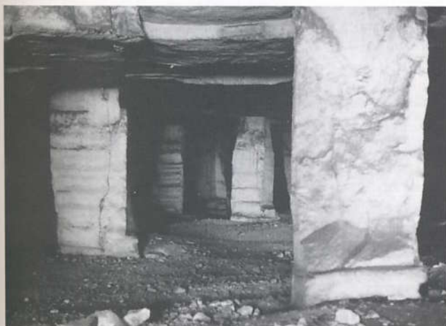
Figure 2.15 Pillars inside an underground limestone quarry at Qau el-Kebir.
