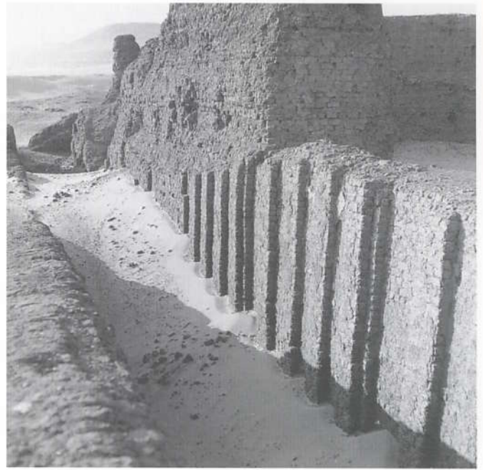
Figure 3.7 Nighed brickwork on the Second-Dynasty 'funerary palace' at Abydos, the Shunet el-Zebib . In the main mass of the brickwork the more pronounced horizontal planes mark layers of grass.
