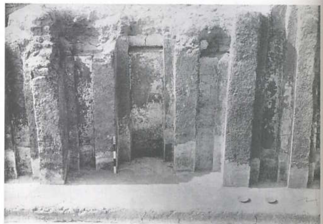
Figure 3.6 Section of niched 'palace-façade' brickwork at First-Dynasty tomb 3507 at Saqqara. Note the impressions of cylindrical wooden poles over the tops of the niches.
