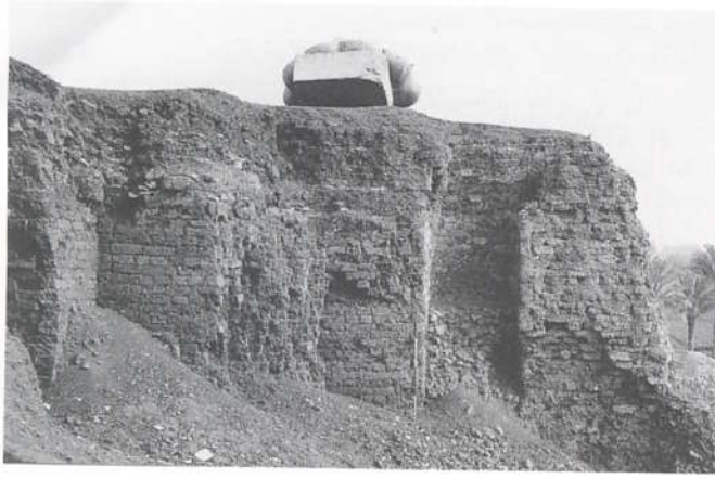
Figure 3.14 Cellular brick foundation platform for the Palace of Apries at Memphis, viewed to the north. The cellular chambers were originally domed.
