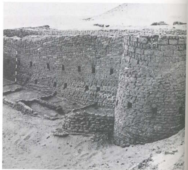
Figure 3.12 Part of the lower ramparts of the Twelfth-Dynasty fortress at Mirgissa, Nubia. Note the angled bedding-planes to take the brickwork uphill.
