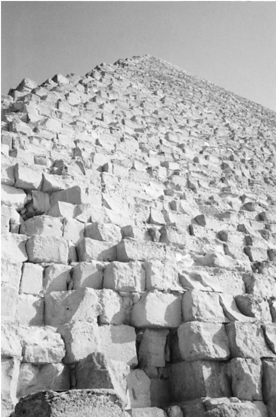
Figure 7.5 Limestone core-blocks in Khufu's pyramid
