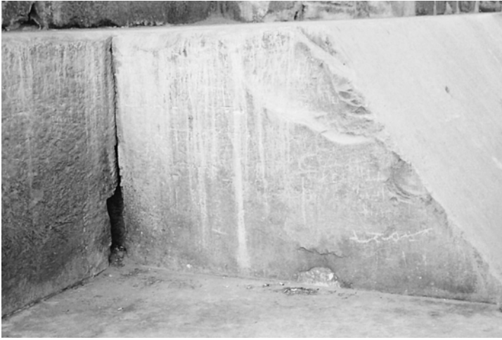
Figure 7.9 The end surface of a casing-block on the northern side of the Great Pyramid
