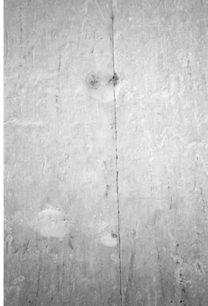
Figure 7.8 Close-up of the rising joint shown in Figure 7.07
