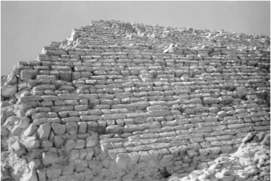
Figure 1.2 Limestone core-blocks in the Step Pyramid, shaped like the mud brick
