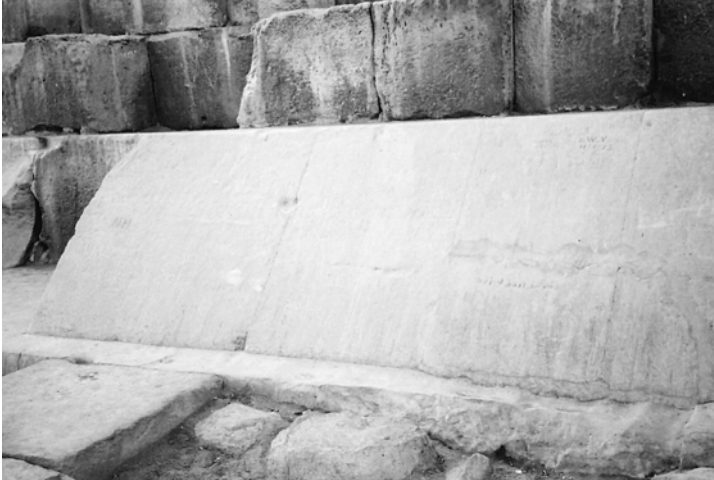
Figure 7.1 Large limestone casing-blocks at the foot of the northern side of the Great Pyramid
