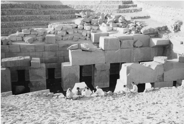
Figure 7.16 Large stone blocks accurately fitted to their supporting pillars in the Osireion at the rear of the temple of Abydos
