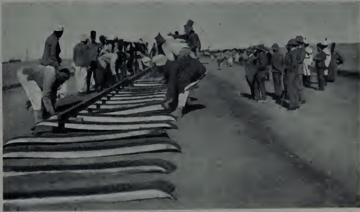
LAYING THE ATBARA-RED SEA RAILWAY.
