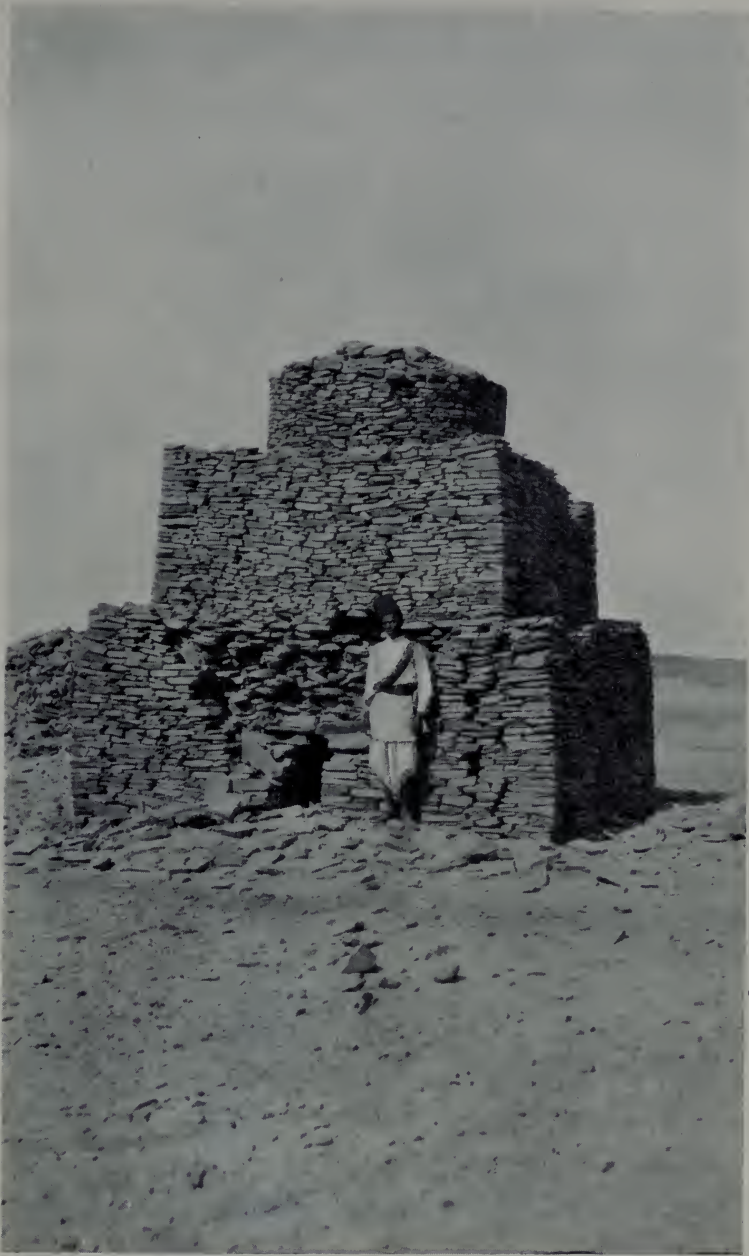
"ANAK" HOUSE AT GEBEL MAMAN ON THE OLD CARAVAN ROAD BETWEEN KASALA AND SAWAKIN.
