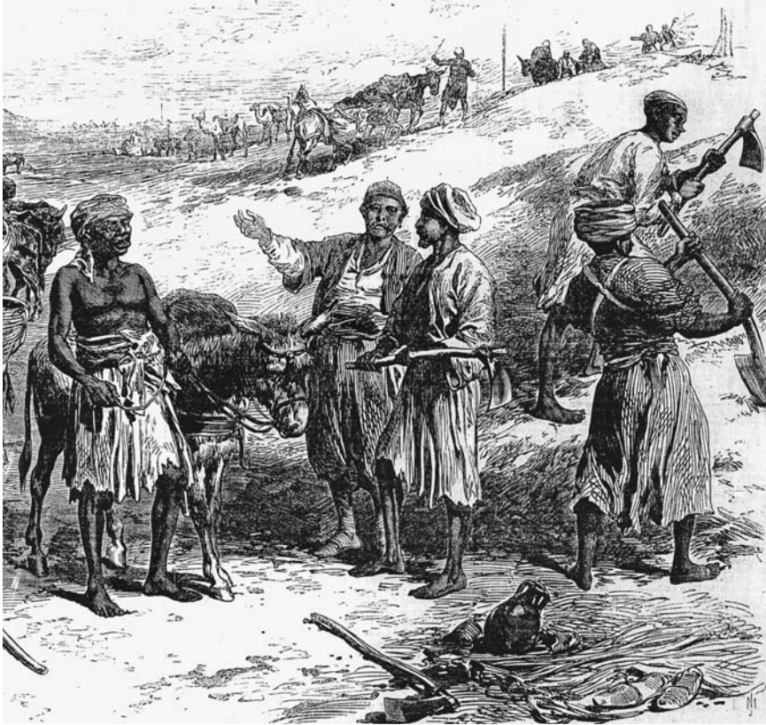
Hired Egyptian workers and their donkeys remove earth from the future bed of the Suez Canal in early 1869. Although dredging machines had replaced unpaid peasant laborers for most excavation work, human labor was still needed as the deadline for completing the canal drew near. (Illustrated London News, March 13, 1869)
