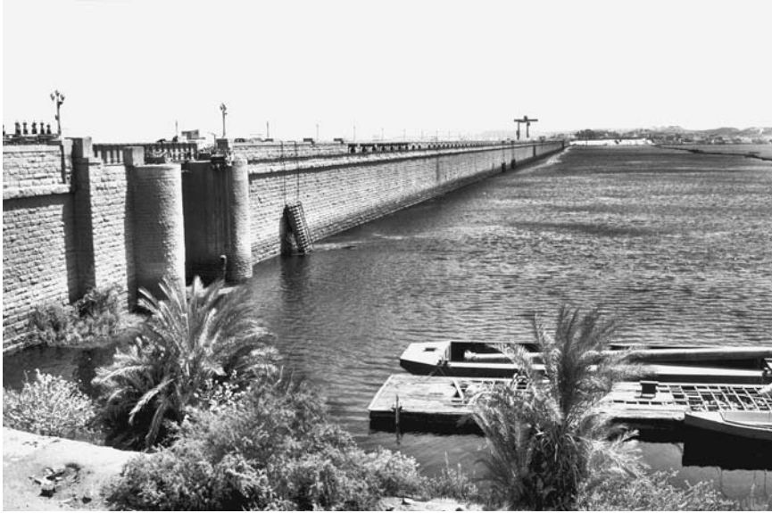
Aswan Dam. Completed in 1902, this dam was enlarged between 1907 and 1912 and then again between 1929 and 1934 to provide water for the perennial irrigation of Upper and Middle Egypt. Its reservoir was never adequate for a high Nile. In 1955 Nasser's government proposed to build the High Dam. (Torben Larsen/Saudi Aramco World/PADIA)
