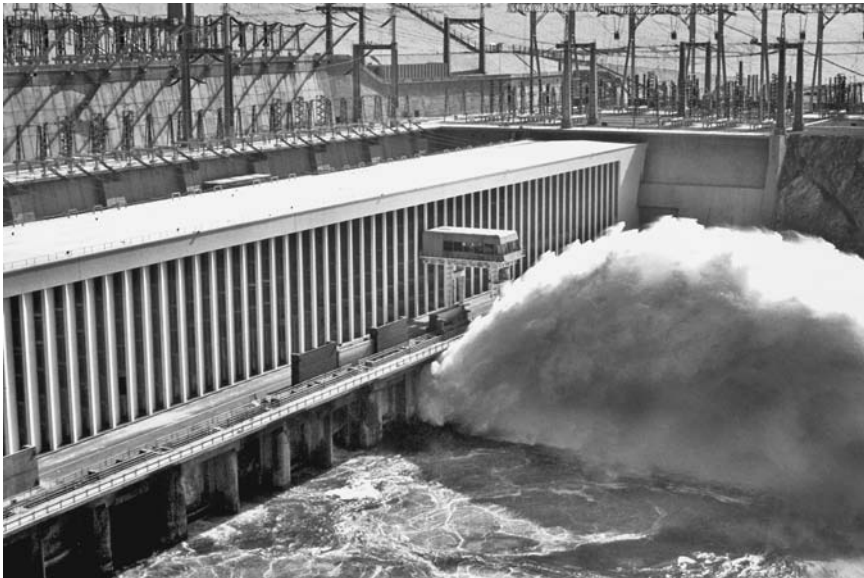
Aswan High Dam. Highly controversial when governments argued in the 1950s over its financing and construction, it was built by Soviet engineers between 1964 and 1971 and has become the linchpin in Egypt's irrigation and electrical power generation. (Tor Eigeland/Saudi Aramco World/PADIA)
