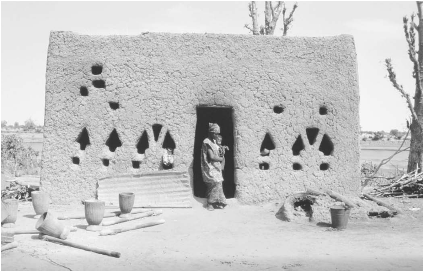
Soninke dried-mud house, with the traditional flat roof and perforated walls. This house, located on the banks of the Senegal River, was photographed in 1988. © Margaret Courtney-Clarke/Corbis
