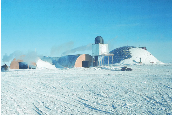
Figure 8.3 South Pole Station after rebuilding in 1975 with a geodesic dome. (Credit: AntarcticaNewZealand)
