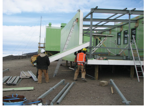
Figure 8.2 Insulation panels in the buildings at Scott Base. (Credit: AntarcticaNewZealand)
