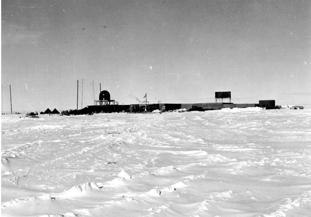
Figure 1.19 The first South Pole Station as it appeared upon completion of construction in January 1957. Snow drift and accumulation eventually buried the buildings, rendering it unusable by the 1970s. (Credit: US Navy, NSF)
