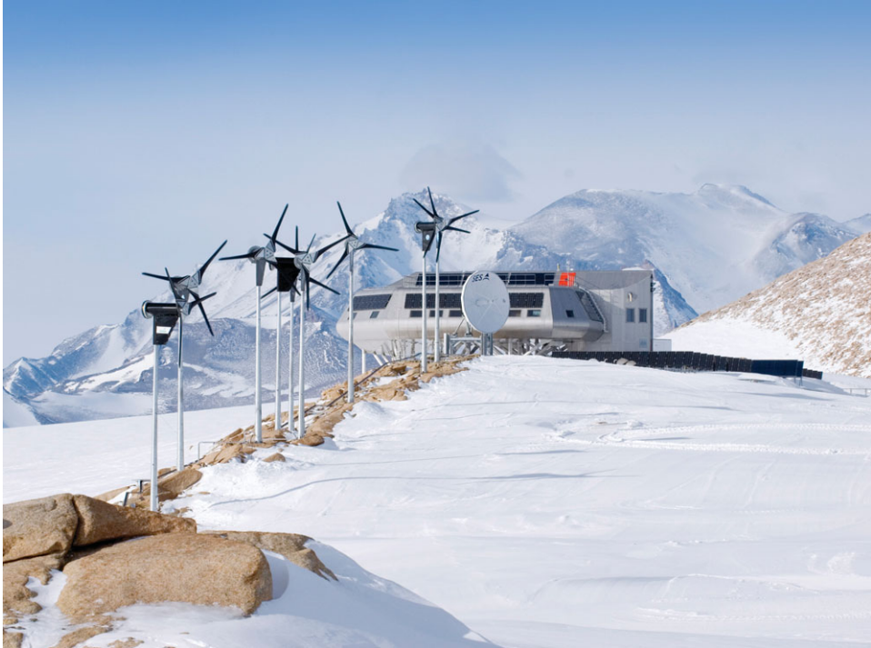
Figure 8.9 Princess Elisabeth station showing the aerodynamic design of the station and the commitment to sustainable energy through wind turbines and solar panels. (Credit: René Robert, International Polar Foundation)
