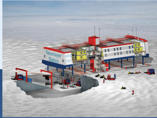
Figure 8.5 (right) Computer graphic of the structure of Neumayer III station showing the hydraulic columns that keep it above the snow surface and the undersnow garage. (Credit: Alfred Wegener Institute for Polar and Marine Research)
