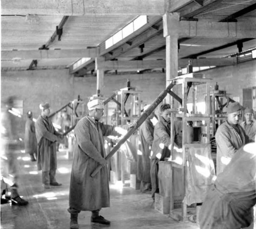
*Plate 21.* View inside the Mine-Filling Factory at Wadi Sarar, with Men Operating Levers to Press Down TNT.
