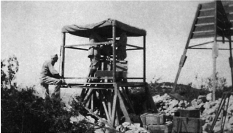
Figure 4.4 Survey post on Jebel Jarmaq (Mount Meron) for the geodetic junction between Palestine and Syria and Lebanon, October 1928 (source: J.H. Mankin photo collection in Palestine Exploration Fund archives, London).
