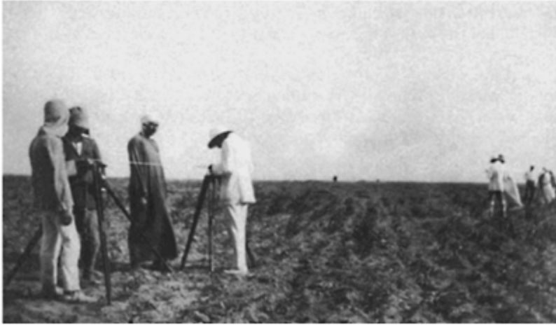
Figure 4.2 Surveyors of the Egyptian Survey Department conducting a check measurement of the triangulation net of the Imara baseline, between points 1'M and 2'M, 1925 (source: J.H.Mankin photo collection in Palestine Exploration Fund archives, London).
