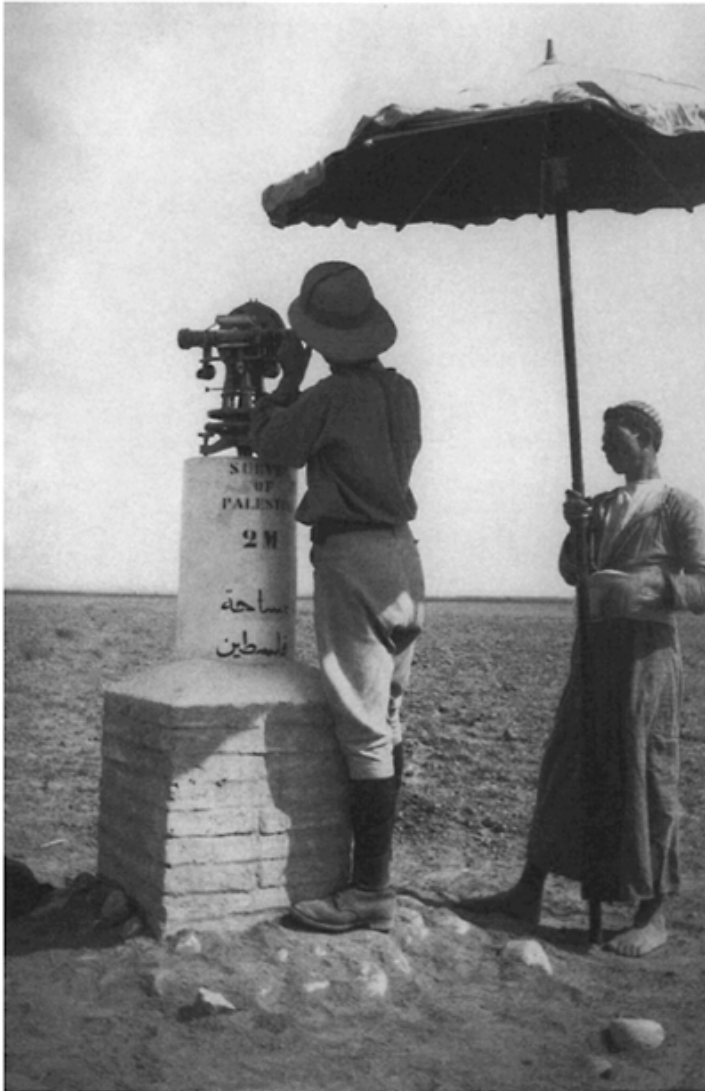
Frontispiece: Measurement taken from point 2'M of the Palestine major triangulation baseline, Imara lands, 1925 (source: J.H.Mankin photo collection in Palestine Exploration Fund archives, London).
