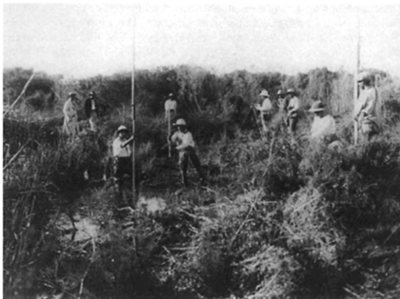
Figure 4.6 Levelling survey in the Kabara swamps, 1925 (source: Photo by Z. Oron–Oroshkes, CZA Subjects/102).
