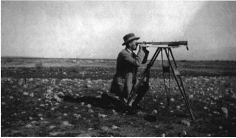
Figure 4.9 The Surveyor John H.Mankin at work with a plane table in the south of the country (source: J.H.Mankin photo collection in Palestine Exploration Fund archives, London).
