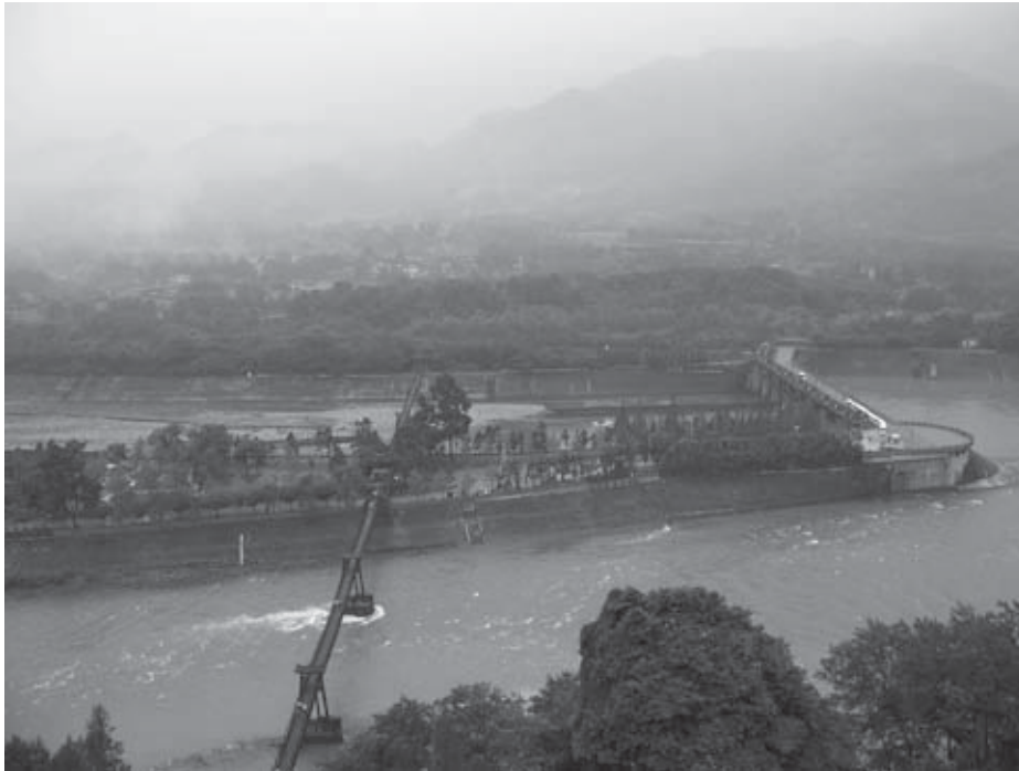
Flooding of the Dujiangyan irrigation system in Chengdu, Sichuan province. PHOTO BY RUTH MOSTERN.
