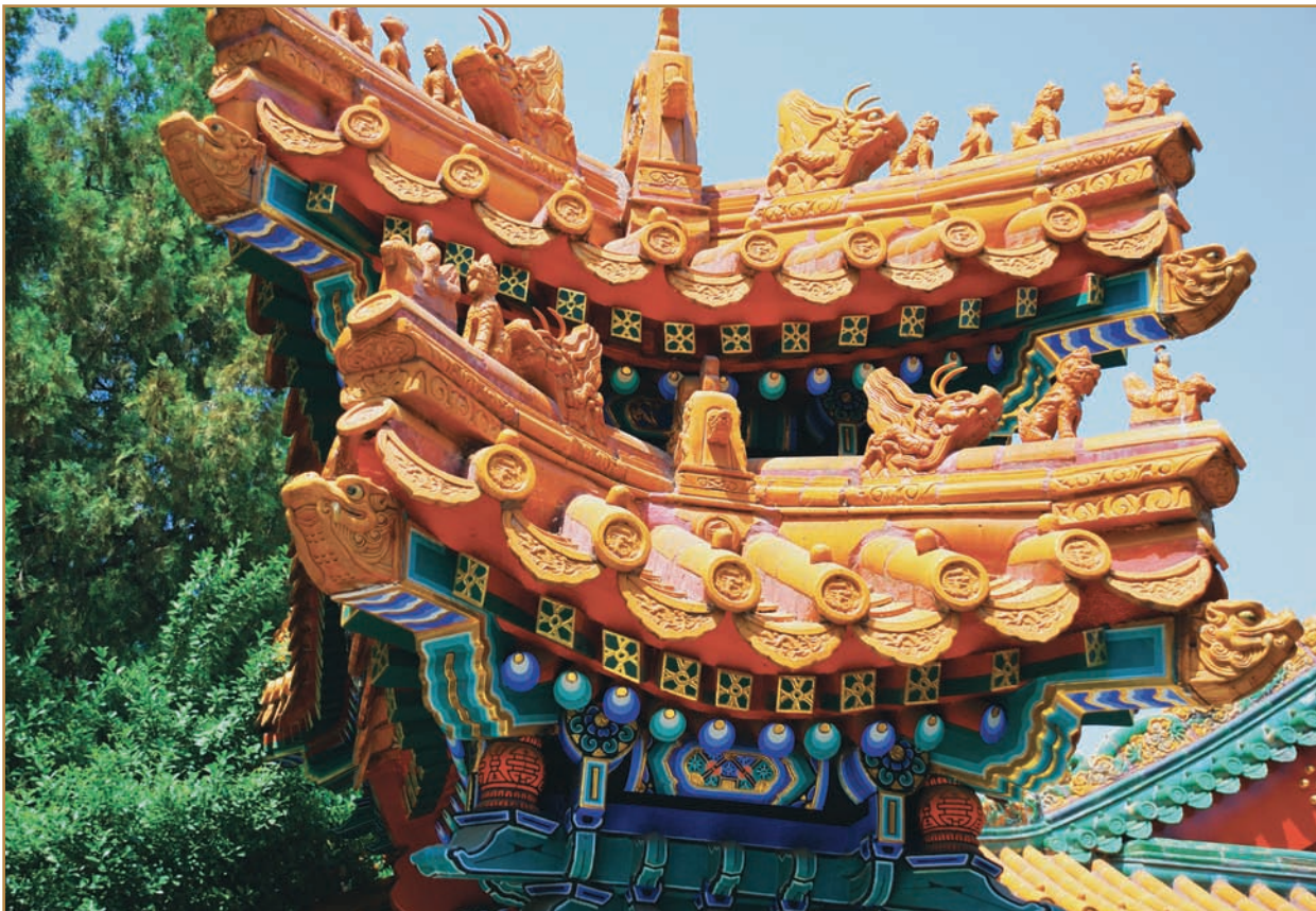
Sculptures of dragons and other mythological creatures are mounted to a building's roof as protection against evil spirits, fire, flood, and other disasters. (Photo by Buchan/Shutterstock)
