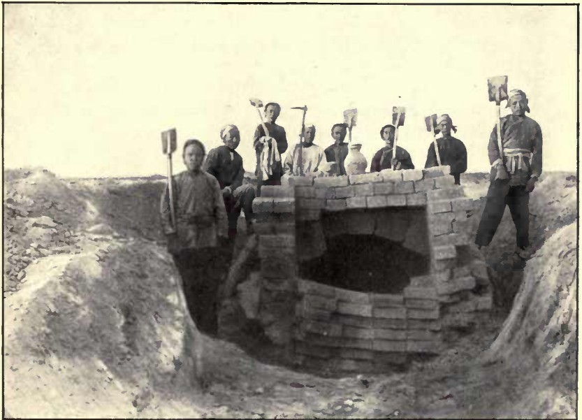
EXCAVATION IN THE DESERT.
