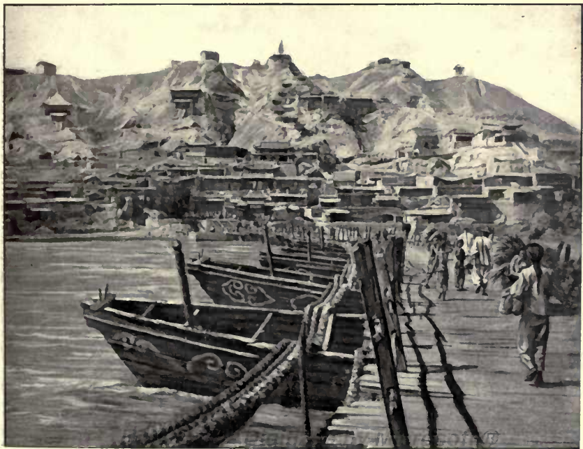
BRIDGE AT LAN-CHU.
