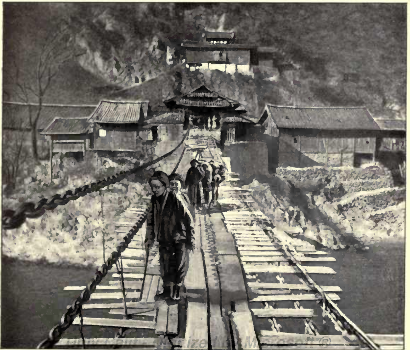
THE BRIDGE OF LU-TING-KIAO.
