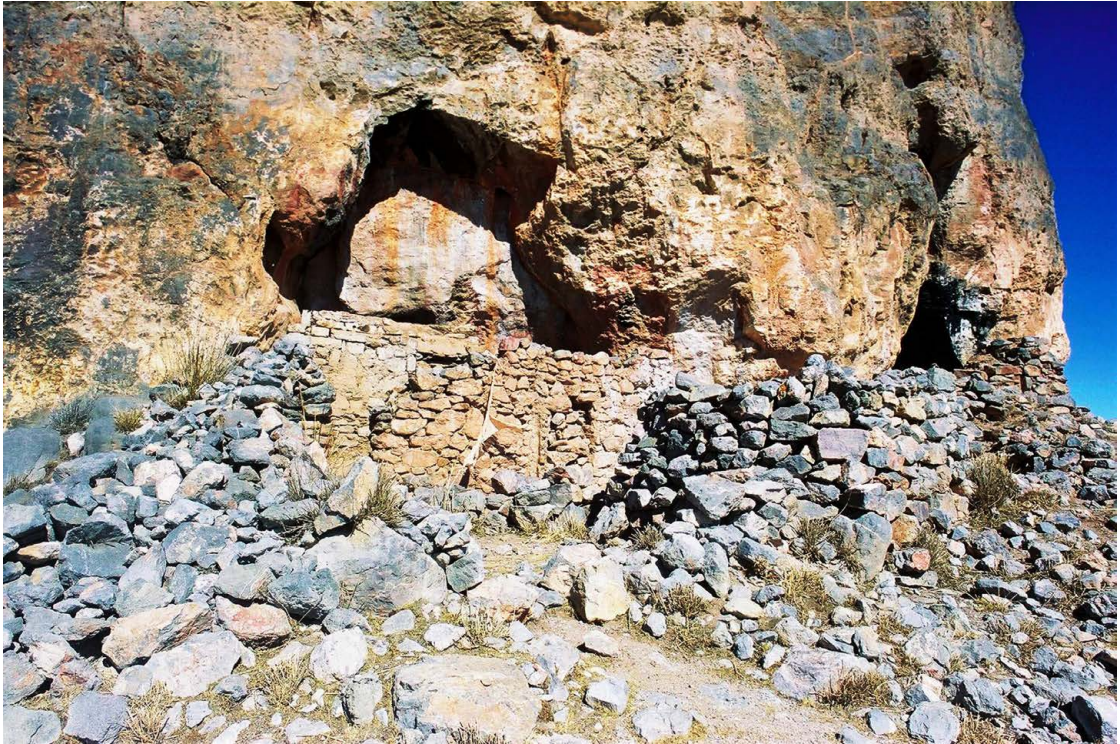
Figure 196. The exterior structures in front of S10_L3.
