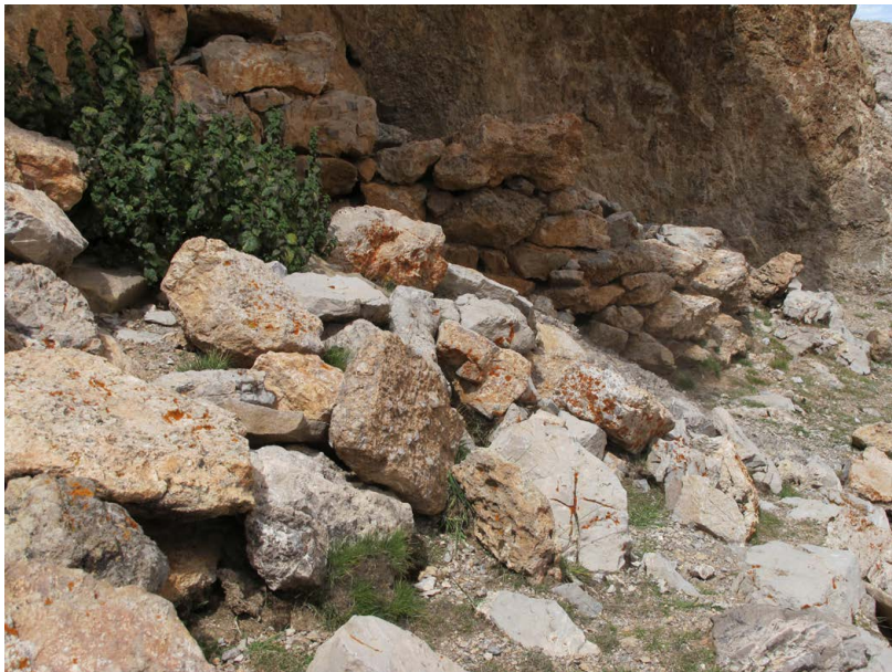
Figure 243. Wall fragments composing part of the forward structural features of S15_L2.
