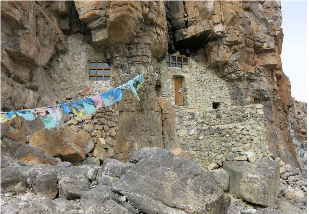
Figure 218. Glang chen phug, Gyer ru mtsho do. As can be seen in the image, the cave is divided into two parts. The right half functioned as a kitchen and fuel storage area and the left (with large window) was used for religious practice and sleeping. The latrine is placed below the kitchen.
