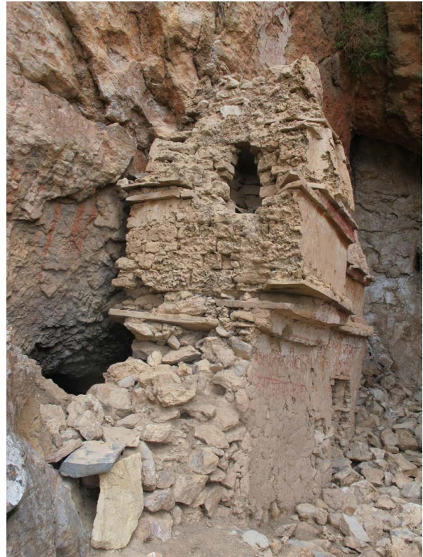
Figure 310. The twin chortens act as a front structure to the recess on the west side of the overhang. A portion of the fire-blackened roof of this sheltered space can be seen at the bottom left side of the image. Note the use of large stone slabs between each main stage of the chorten .
