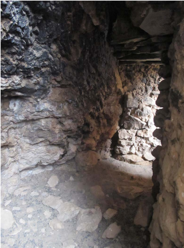
Figure 311. The interior of the chamber. The entranceway to this sheltered space via the north member of the twin chortens is visible in the background. Note the corbelled stone ceiling.
