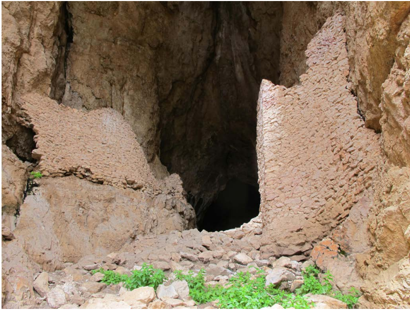
Figure 295. Massive masonry walls set inside the forward portion of Sgar gsol brag phug (S27).
