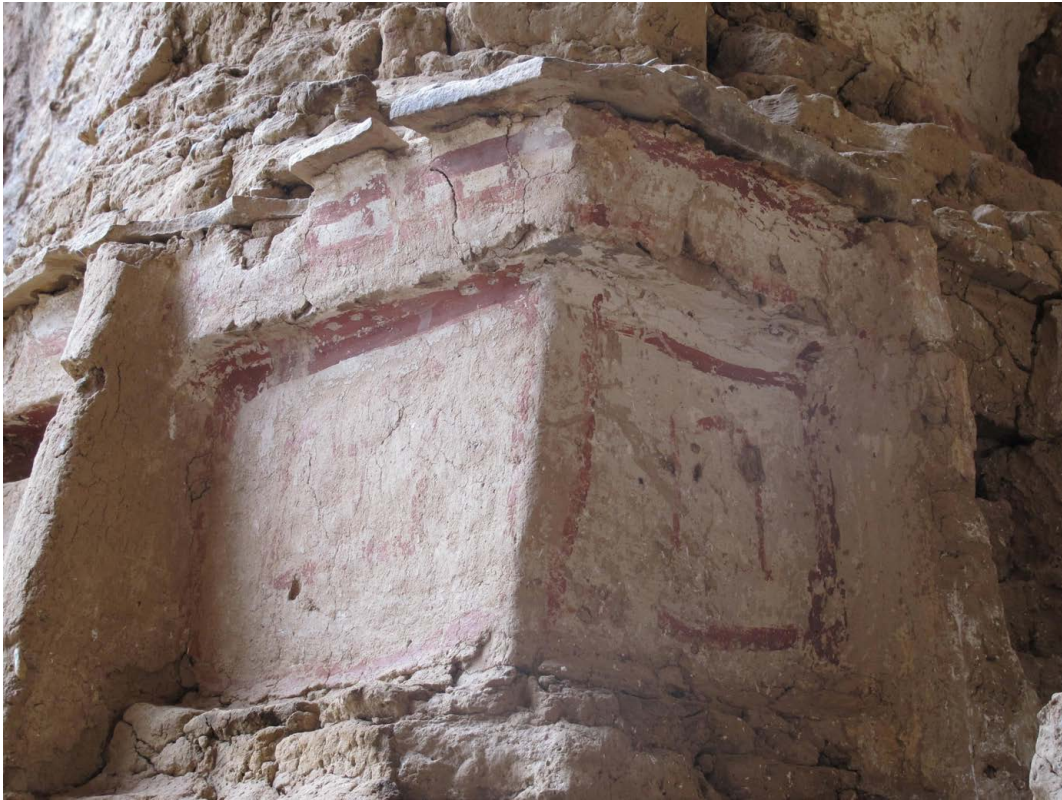
Figure 306. Traces of what appear to be the original embellishment of one of the chortens , made with red, yellow, and white mineral pigments.
