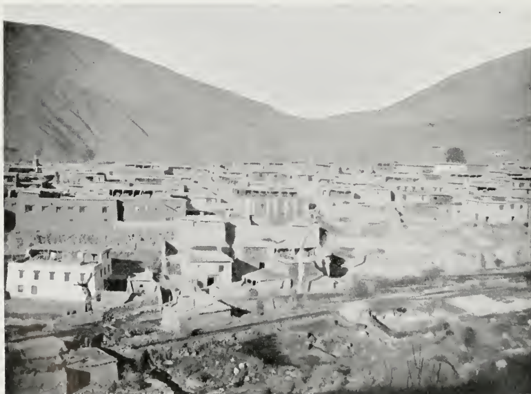
BATANG, LOOKING NORTH
