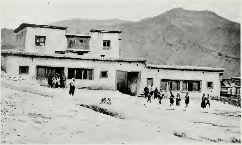
OFFICIAL'S HOUSE AT DRAYA JYAMDUN
