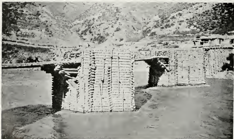
THE "SZECHUAN BRIDGE" ACROSS THE DZA CHU AT CHAMDO
