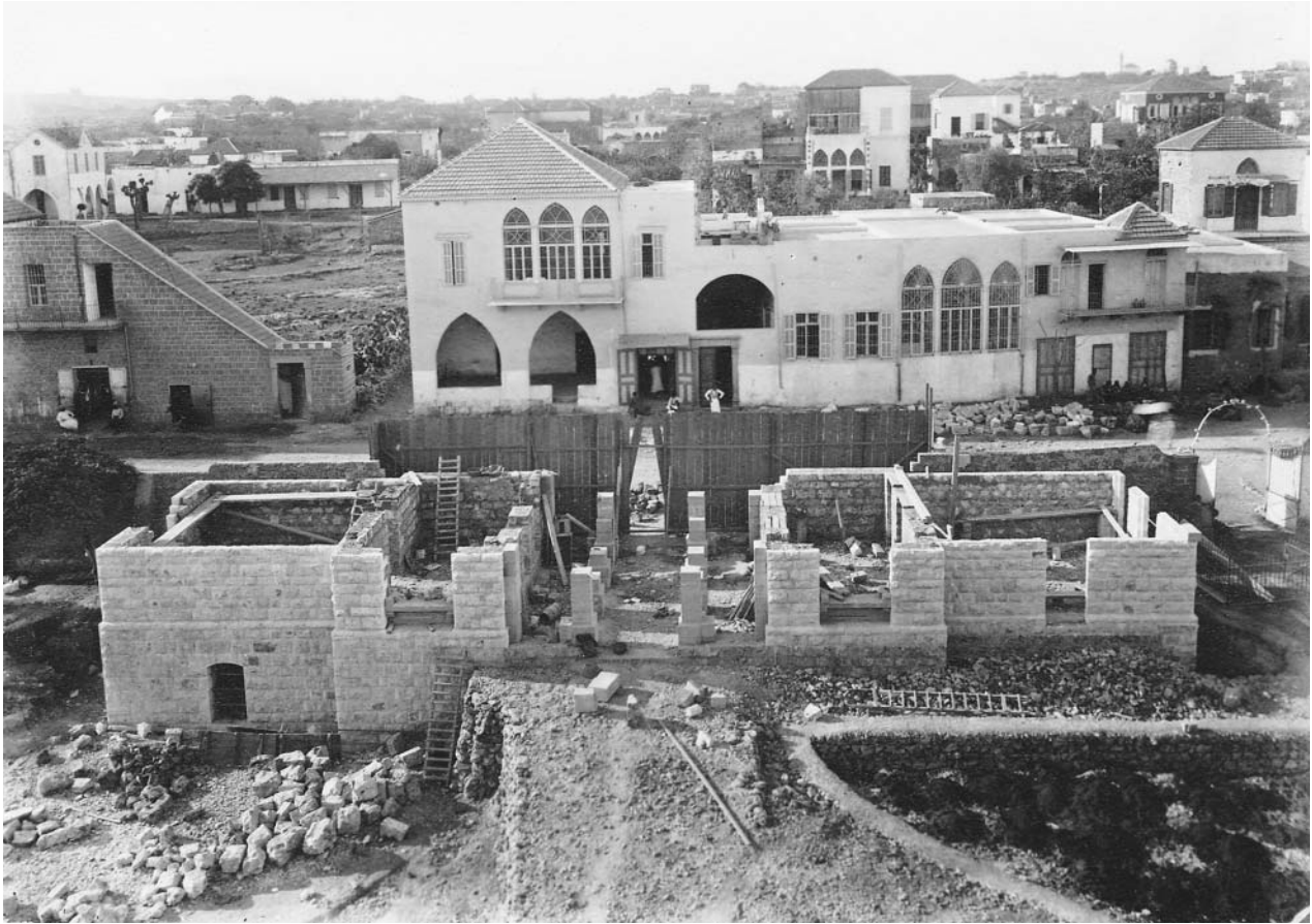
A missionary school under construction. © AUB ARCHIVES. REPRODUCED BY PERMISSION.
