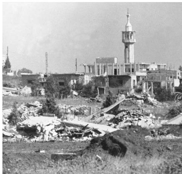
The town of Qunaytra in the Golan Heights was destroyed by Israeli forces during the Arab-Israel War of 1973, an act that later led to a United Nations accusation against Israel for violating the Geneva Convention. After the war, the Syrians refused to rebuild and reoccupy Qunaytra, insisting rather that the flattened remains stand as mute testimony to what they consider Israeli brutality. © AP/WIDE WORLD. REPRODUCED BY PERMISSION.
