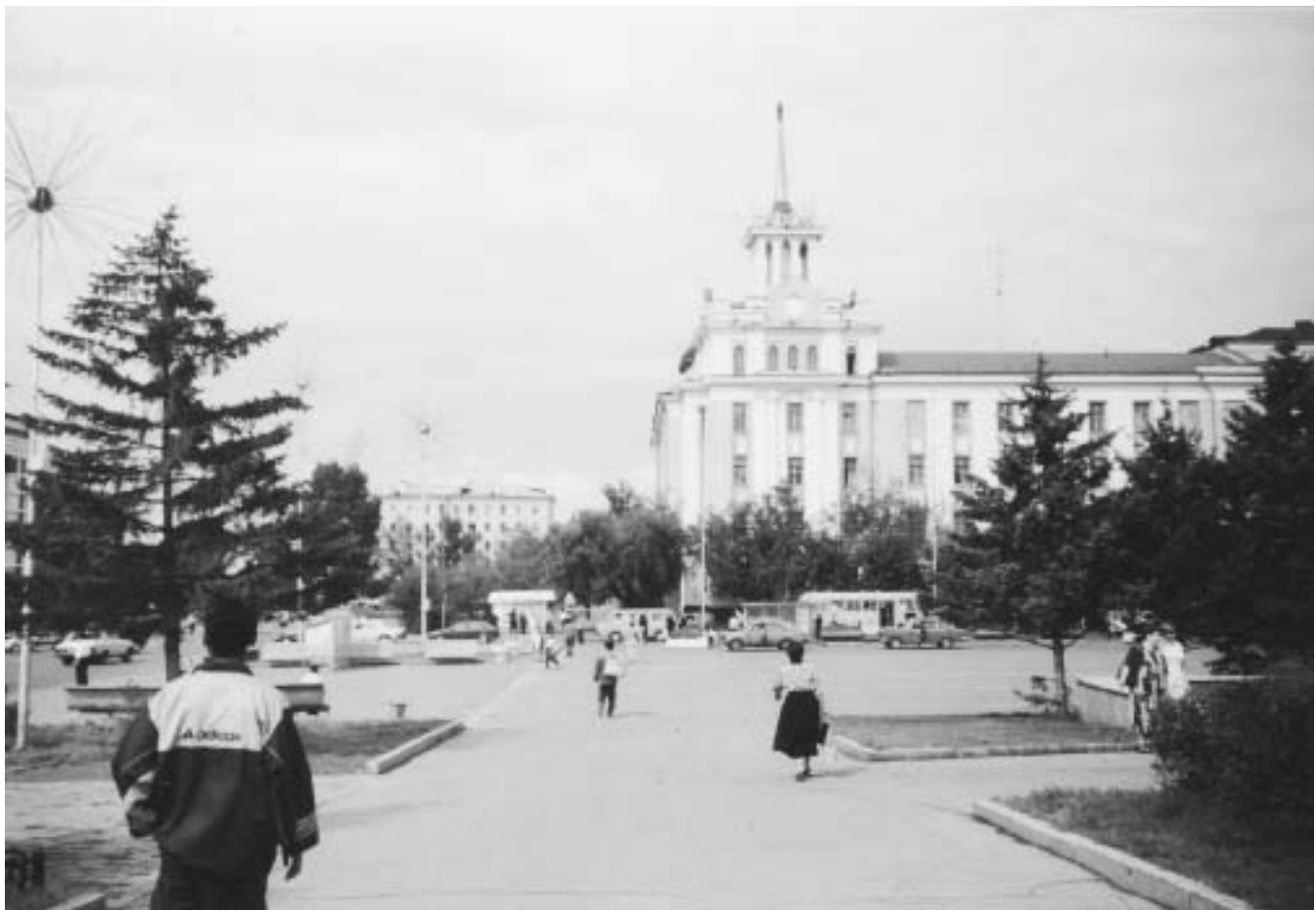
Buriat Radio and Television Building near the Central Square of the Soviets, Ulan-Ude (Courtesy Tristra Newyear)
